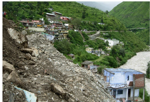
Figure 2. Photograph of an active landslide in the study area damaging number of houses, part of the road, agriculture land and infrastructure (14 August, 2010)
