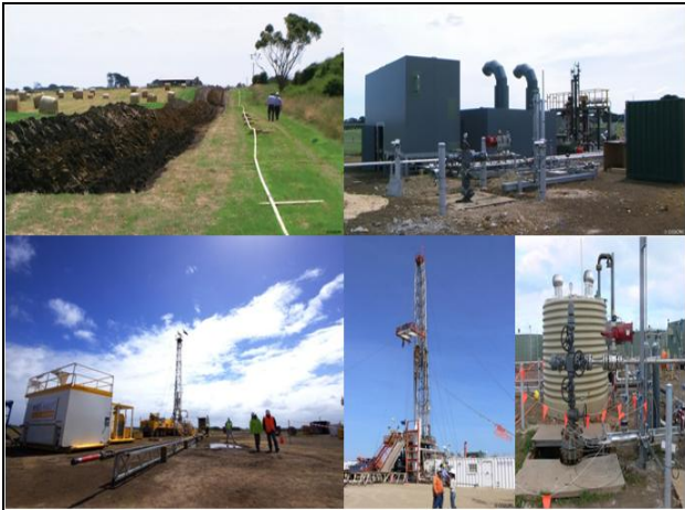
Figure 2. Execution phase at Otway CO2CRC
