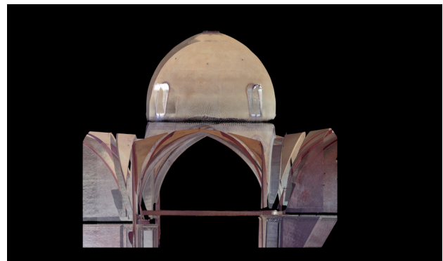
Figure 7. Image of the point-cloud of the intrados of the Basilica's dome.
