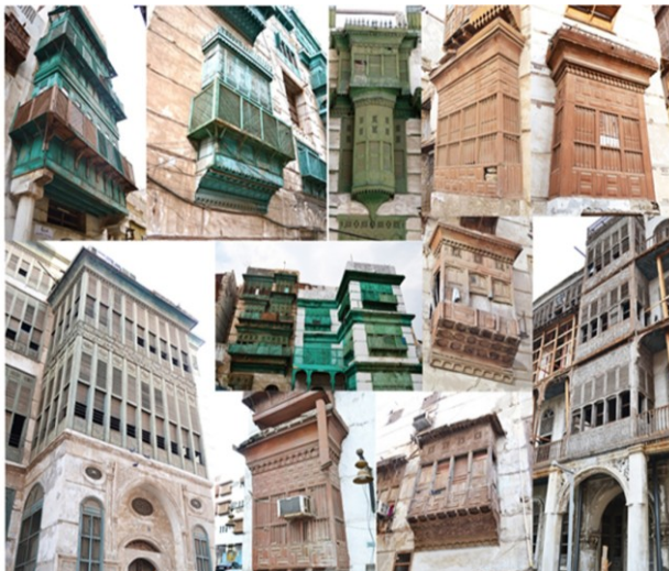
Figure 1. Examples of different types of Roshans in the Historical City of Jeddah.
