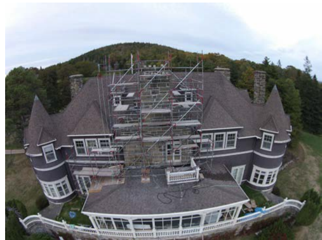
Fig.4 – Roof details captured with the UAV
