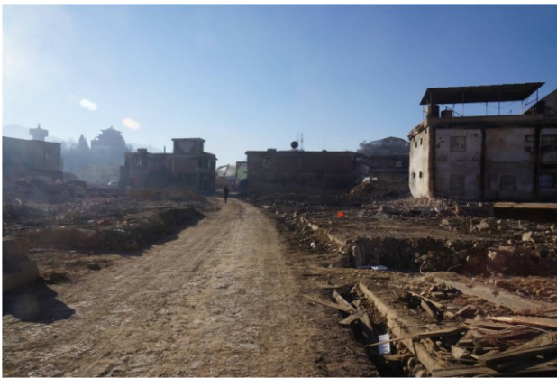
Figure 3. North Gate Street After the Fire Photo: Dr. Ing. HUO Xiaowei
