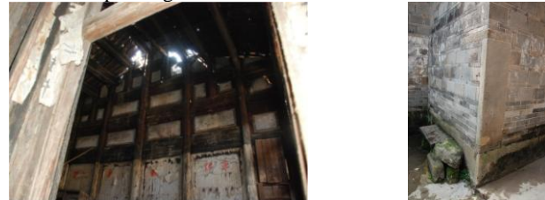
Figure 8. Pictures of the building structure and the rowlock wall
