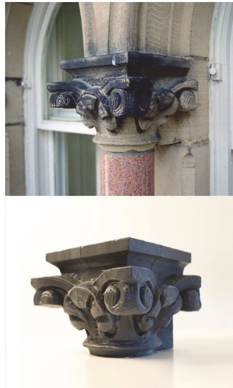
Figure 3. Pilaster capital (top) and 1:1 3D-printed capital maquette (bottom)
