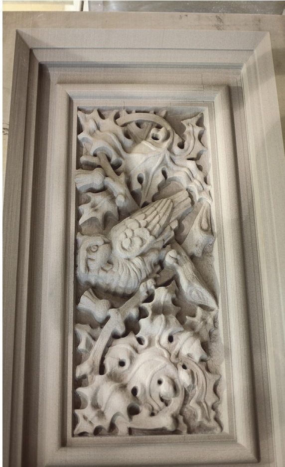
Figure 9. Robotically milled sandstone relief sculpture, prior to hand-applied finish
