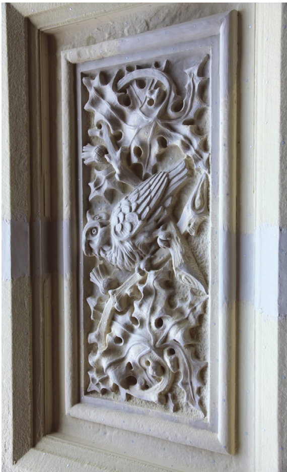
Figure 7. CNC-milled polyurethane foam maquette of relief sculpture with modelling clay applied
