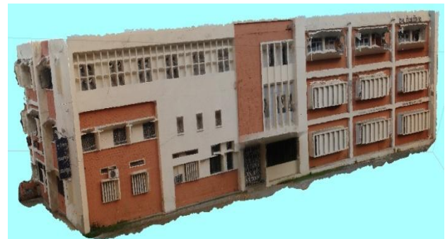
Figure 14: Textured 3D model of transportation section at civil engineering department
