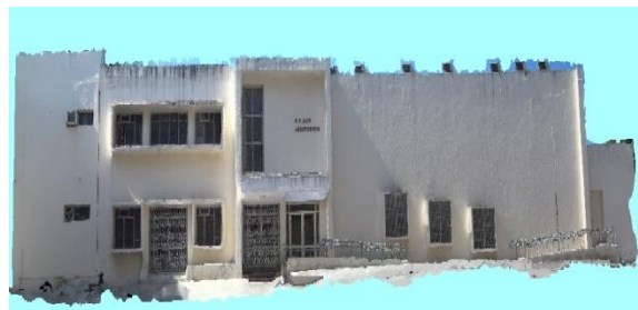
Figure 12: Textured 3D model of O.P.Jain auditorium building of civil engineering department
