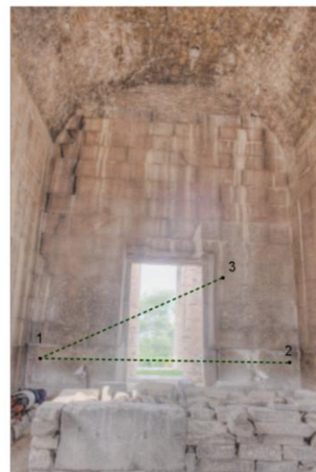
Figure 9: The three geodetically measured points
