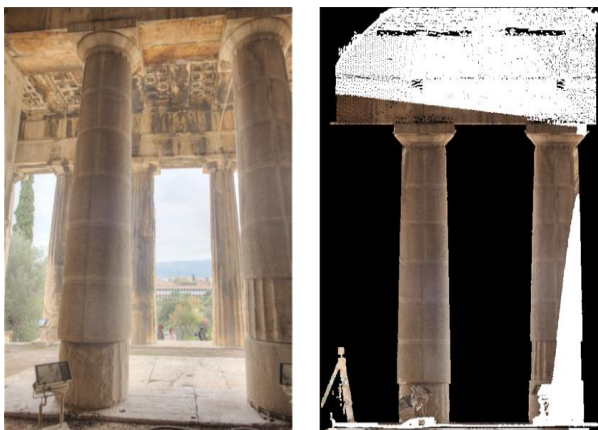
Figure 11: Left: Oblique image of the east interior entrance that used in the algorithm. Right: The produced orthophoto
