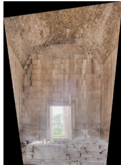
Figure 8: Final georeferenced image through rectification
