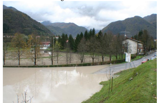
Figure 8. Flood in Tolmin on 5 November 2012 (photo: R. Lipušček).
