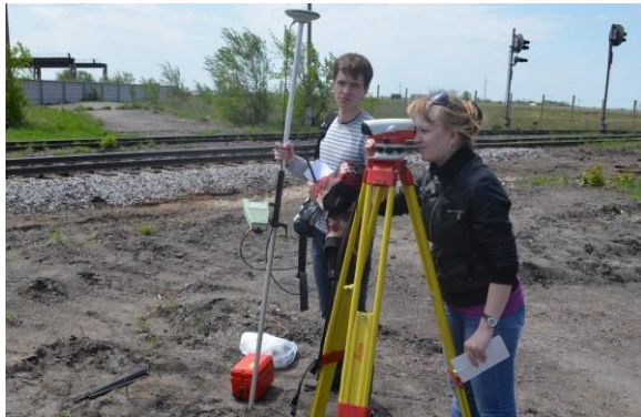
Figure 2. Carrying out of a ground monitoring
