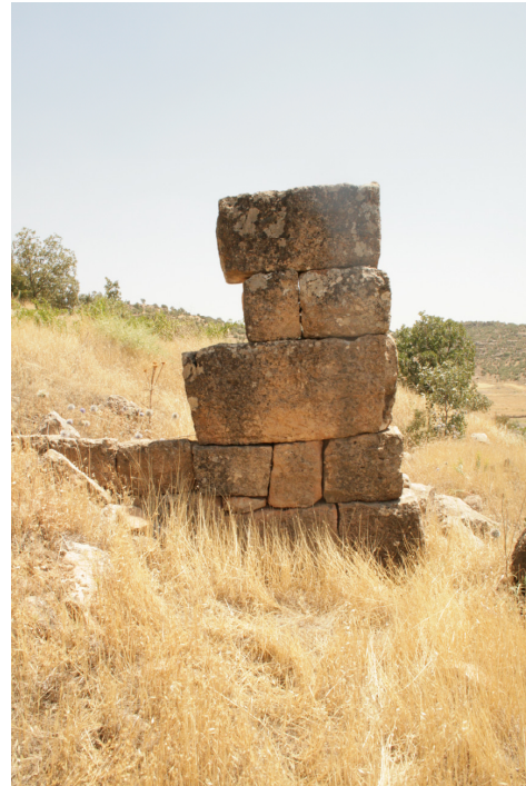
Fig. 7. Keferde, the wall on the southwestern slope with a corner showing trapezoidal masonry technique. View from the W. Photo: Minna Silver 2016.
