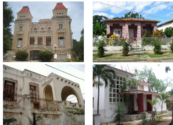
Figure 2. Examples of Vista Alegre’s architectural collection. Note the integration of green areas. Source: authors’ archives
