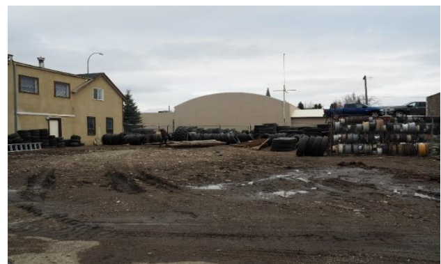
Figure 10: The Quon Sang Lung Laundry building site following demolition of the structure. Source: Peter Dawson
