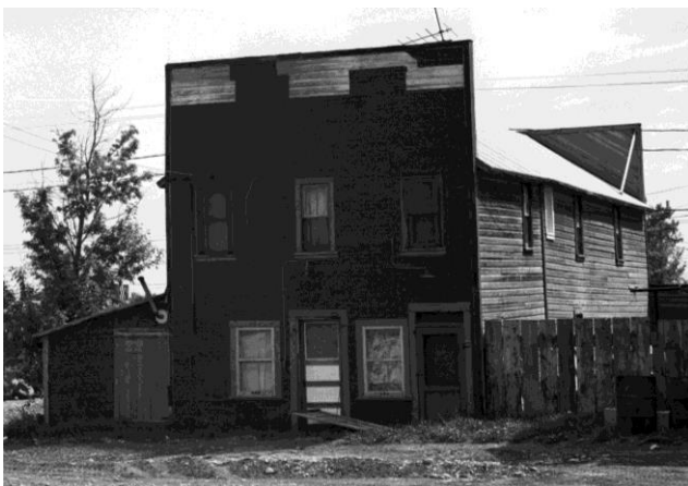
Figure 2: Addition at rear façade with boomtown storefront addressing 25 Street; shed at east side; Insulbrick cladding, regular fenestration pattern, (2) entrances, 1973. Source: HRM
