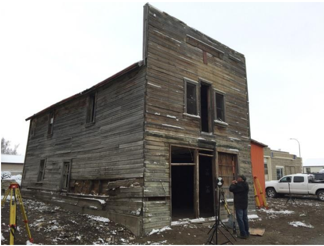
Figure 4: South and west facades. November, 2016.
