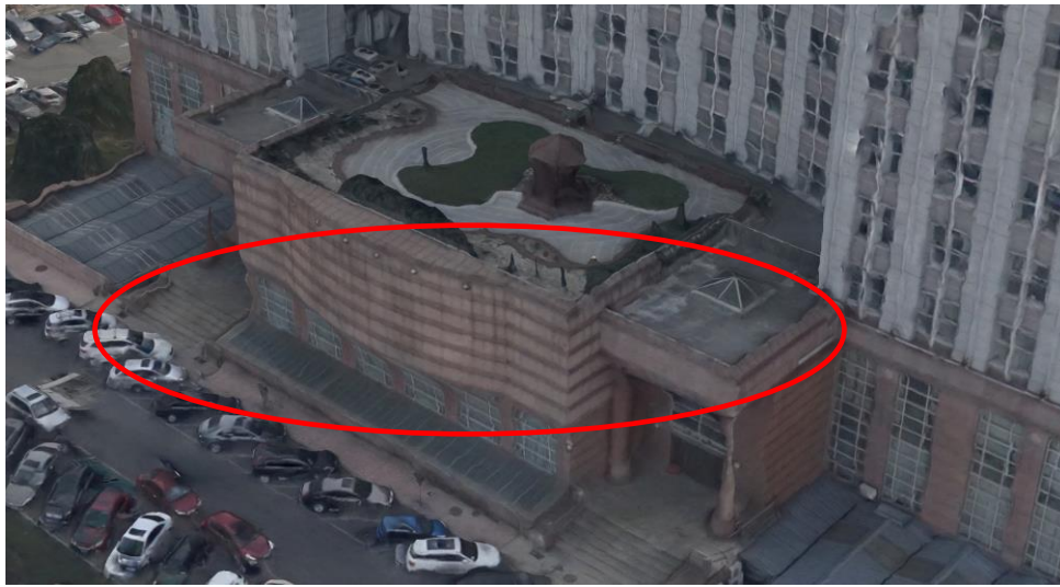
Figure 12 The air view of one big building model produced by OP only
