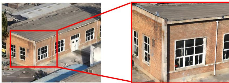
Figure 8 The model constructed by the oblique photogrammetry and the ground photogrammetry
