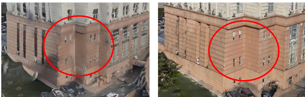
Figure. 11 The side of one building model produced by oblique photogrammetry(OP) only(left) and produced by OP and
