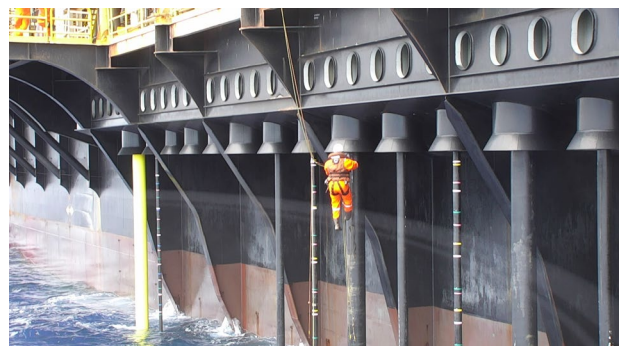
Figure 1. Industrial climbing for riser inspection.
