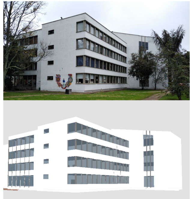
Figure 6. South-West side of the building
