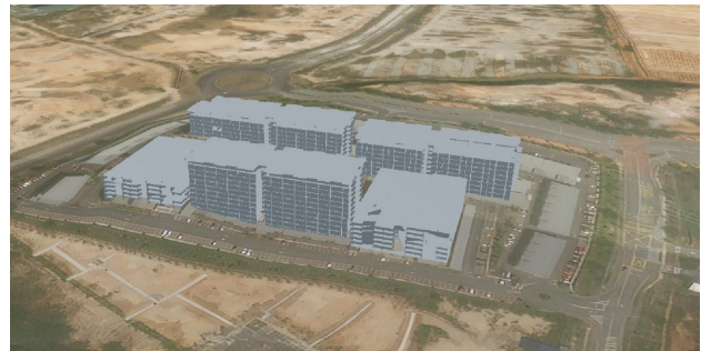
Figure 5. The scheme of 12778 converted from Strata XML to CityGML with Strata ADE. Visualized in SKiP portal.
