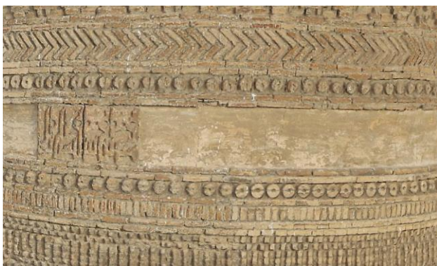
Figure 10. Detail of Kalon Minaret from the 3D model showing missing parts. Source: authors.
