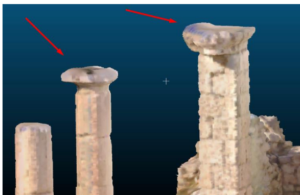
Figure 13. Deformations (little swollen) on the column capitals.
