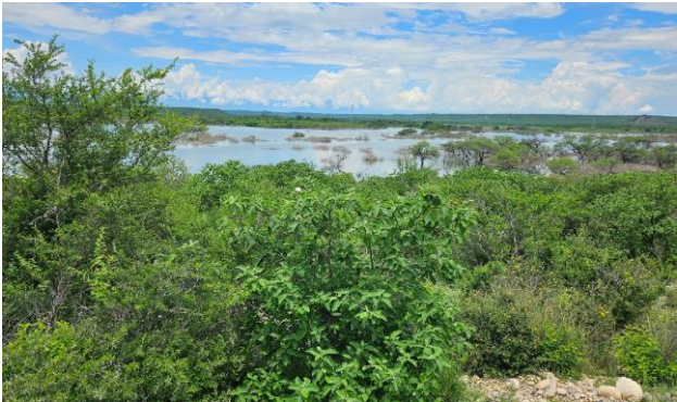
Figure 7. La Libertad dam and some vegetated areas flooded.
