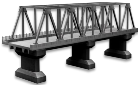
Figure 10. Truss bridge (height: 30.4m length: 100m width: 22.1m)
