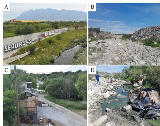
Fig. 8. Different problems were recorded with ground-level photos. A) This photograph shows a concrete channel used for river drainage, the wall of which is covered in graffiti, reflecting a possible lack of maintenance and surveillance in the area. Photograph taken from a bridge. B) In this ground-level image, accumulated waste is observed on the riverbed; this accumulation was analyzed using a point cloud. C) On the banks of the Pesquería River, it is common to identify homes that are located within the floodplain; these are usually irregular homes that are not legally registered. Photograph taken from a bridge. D) In this image, accumulations of solid waste are observed on the riverbed; this scene is constant in different areas of the main channel.
