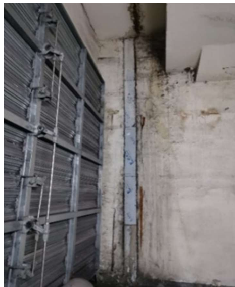
Figure 1. Case of underground engineering leakage.
