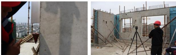
**Figure 2.** Verticality check of using traditional manual measurement (left) and using laser scanning approach (right).
