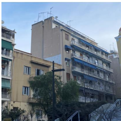
Figure 3: Small terrace surface area and unbalanced building heights Eratosthenous str, Athens Greece (Source: authors editing)
