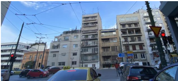
Figure 2: Unbalanced building heights on King Constantine Avenue, Athens, Greece (Source: authors editing)
