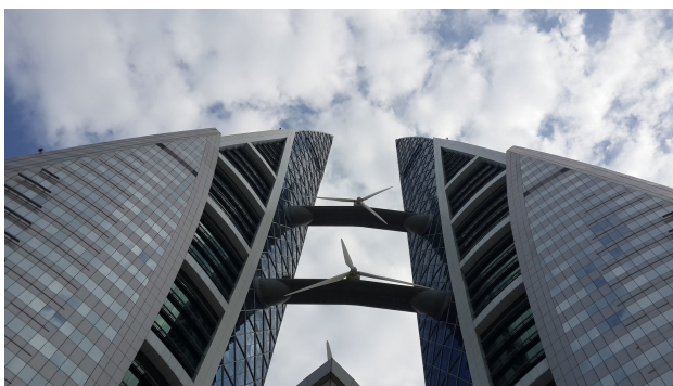
Figure 1. An array of three wind turbines is integrated between the two towers of the Bahrain World Trade Center (by Denise Krebs is licensed with CC BY 2.0).
