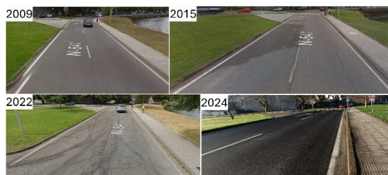
Figure 2. Visual images overtime on the road section.
