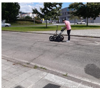
Figure 10. Data collection and GPR-GPS system setup.
