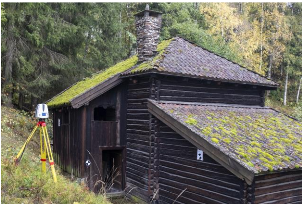
Figure 3. The log house and the Leica P40 scanner
