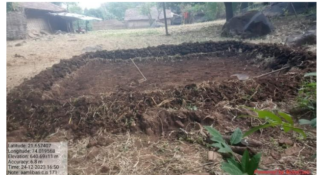
Figure 2. Field view of a Jalkund rainwater harvesting structure implemented in the Molgi cluster for localized moisture retention
