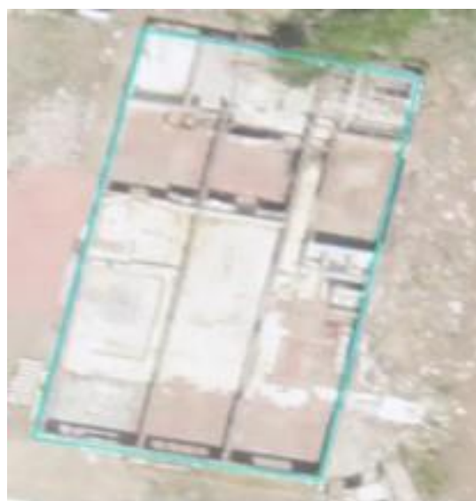
Figure 6. Completely damaged building misclassified as partially damaged. Although elevation attributes correctly classified it, using texture attributes led to misclassification due to conflicting cues.
