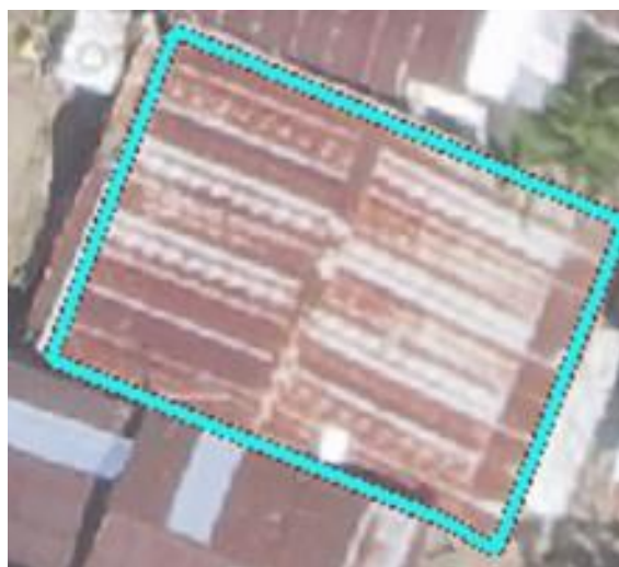
Figure 4. Building with roof made of rusted corrugated sheets. The rusted and uneven texture of the roofing material introduced noise in the texture attributes, leading to frequent misclassification as damaged despite being intact.
