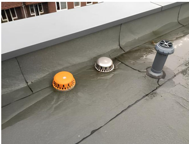
(a) drainage outlets for rainwater and ventilation for flat rooftops Hagmans GmbH 1
