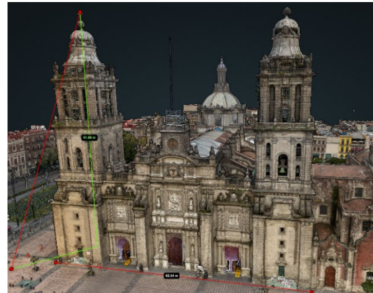
Figure 3. Mexico City Metropolitan Cathedral photogrammetric model.
