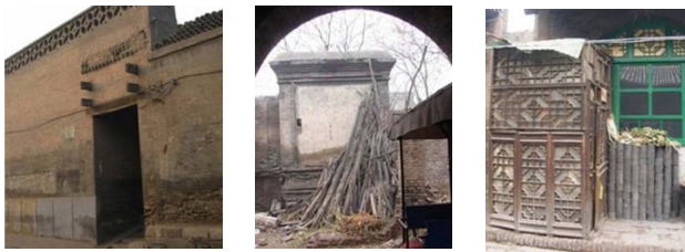
Figure 10. Poor living conditions in Pingyao before (Source: same as Figure 5)
