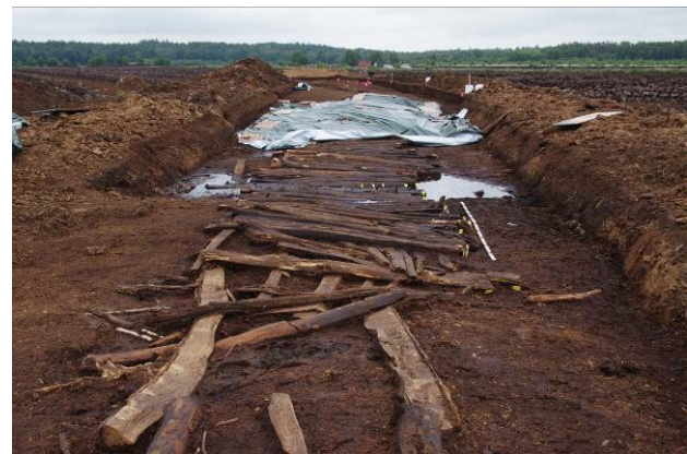
Figure 3. Zone 2 lower construction and zone 3 upper construction (C. Melisch, 2019)
