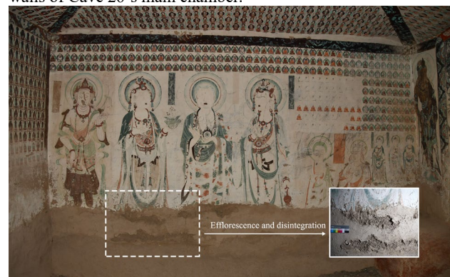
Figure 6. Efflorescence and disintegration on the south wall of the main chamber of cave 26 of Mogao grottoes.
