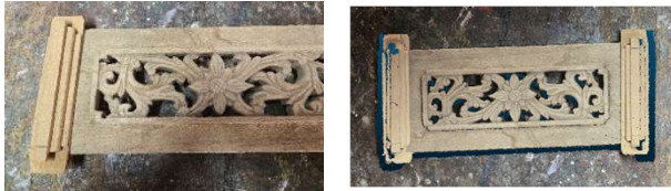
Figure 11. Carving Integrated with Concealed Tenon (Photograph on the Left, Point Cloud Data on the Right)
