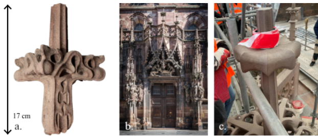
Figure 4. a) Photograph of the sculpted artifact; b) Saint-Lawrence portal, Strasbourg's Cathedral, France © Claude Truong-Ngoc 2020; c) Typical case for very close range photogrammetry on scaffolding, Heritage restoration site of Saint-Lawrence portal's. Photo courtesy and © G. Calmels 2025.
