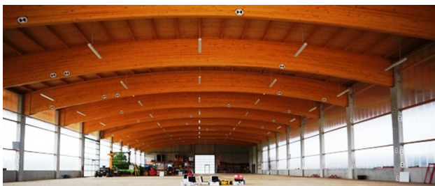
Figure 1. Used Facility to determine CPs containing planar structures and TLS targets in an optimized geometry introduced by Medić et al. (2019b).
