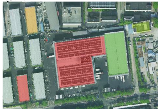
Figure11.High-risk building optical images
