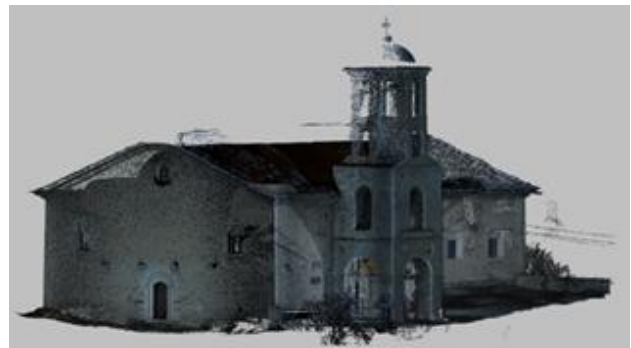
Figure 6. TLS-derived point cloud of the exterior of the Church of St. Petka.
